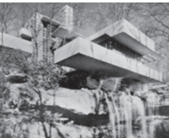
SL. 7. Frank Lloyd Wright: Fallingwater House, Bear Run, 1936.
