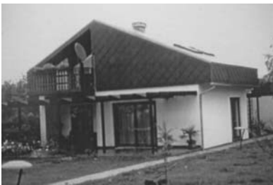
Slika 4: Kuća u Ivanić-Gradu prije obnove i dogradnje House in Ivanić-Grad before refurbishment and extension.
